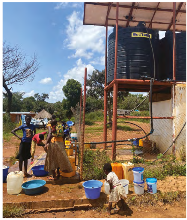
© ↑ Water borehole built by Kamoa in Muvunda, 26 February 2022 © Amnesty International (photographer: Candy Ofime)
